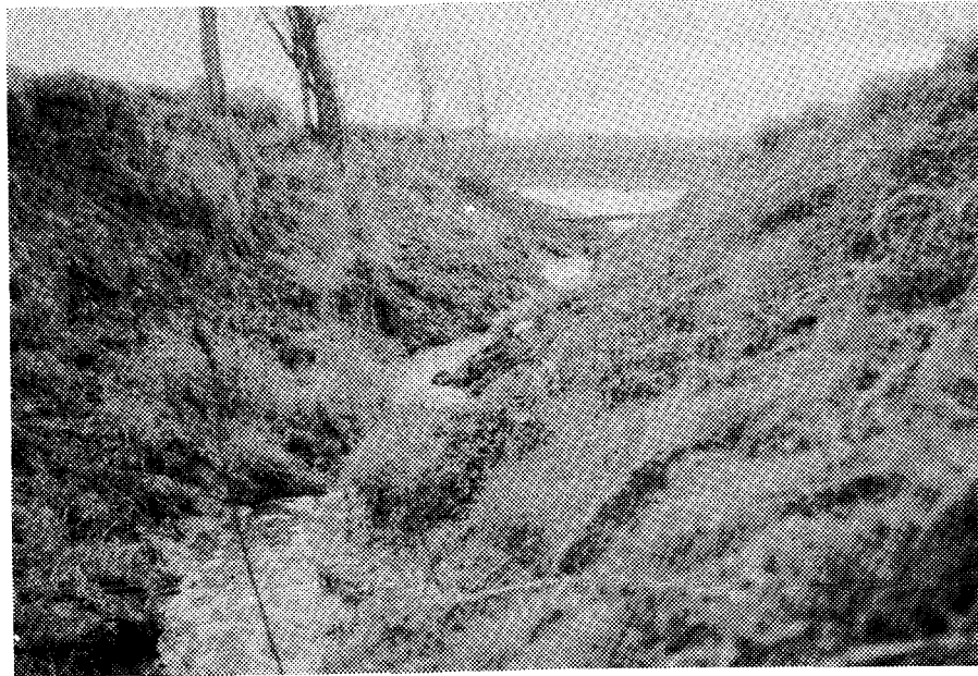
PHOTO 3.3.3 POORLY CONSTRUCTED DRAIN
