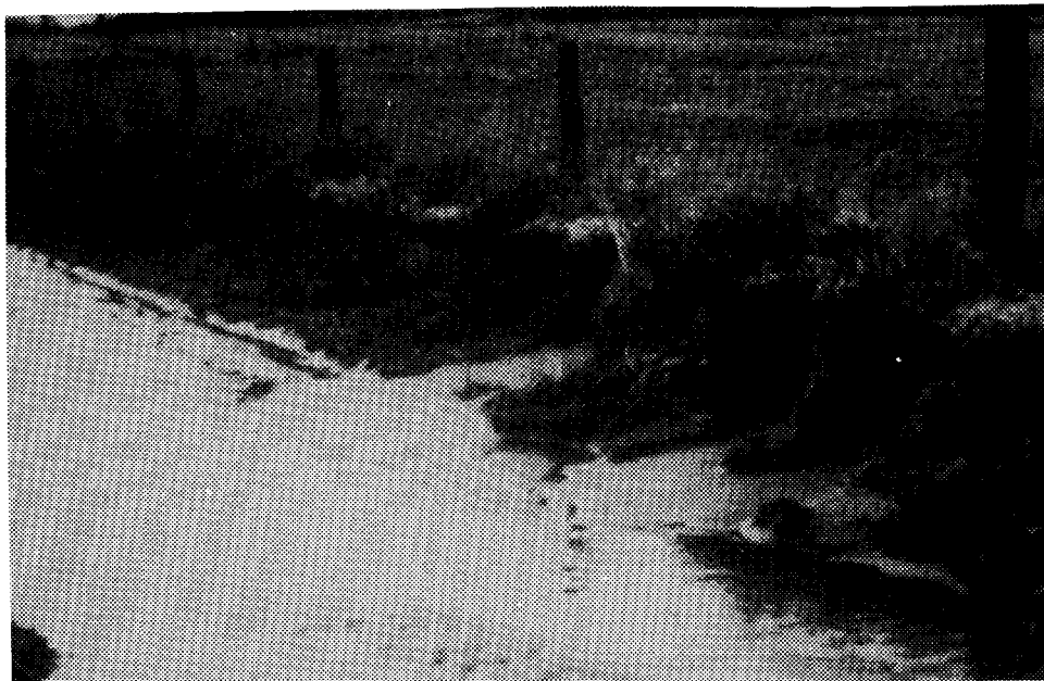
PHOTO 3.3.4 DRAIN SHOWING EROSIONAL DAMAGE
