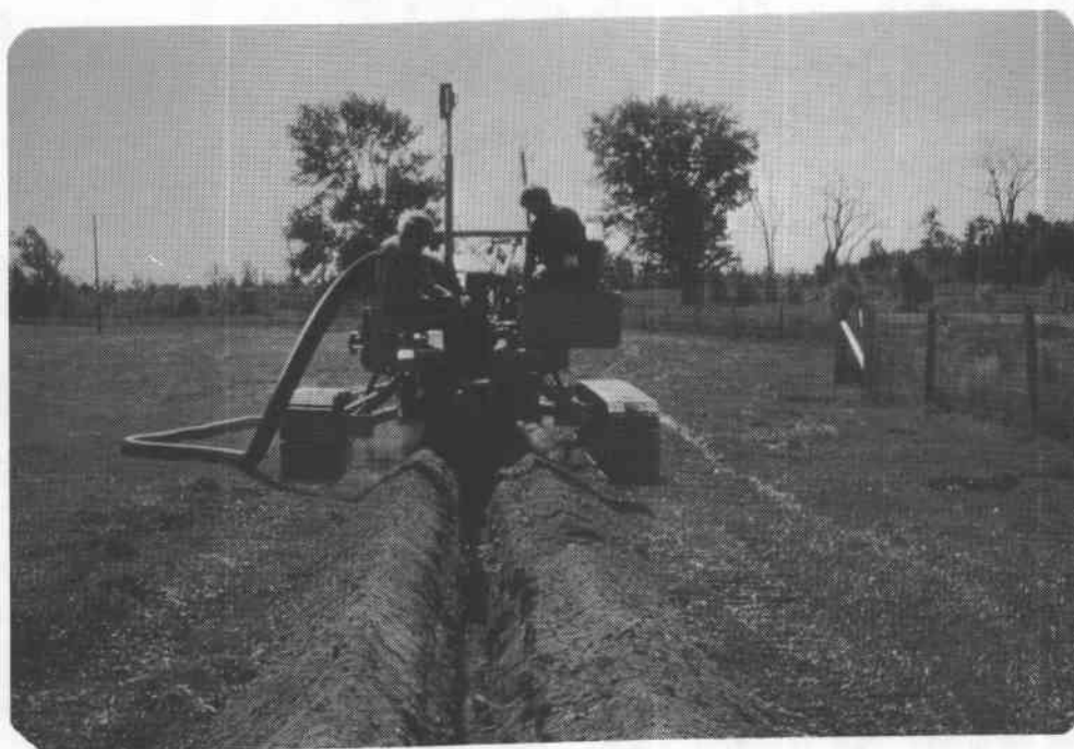
PHOTO 2.2.6 INSTALLATION OF TILE DRAINS
